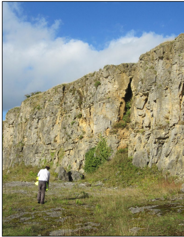
A marked cavity in the face, NE corner.
