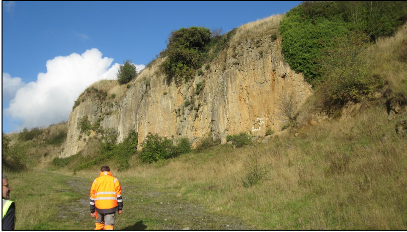
Karstified face at southern end, upper bench.
