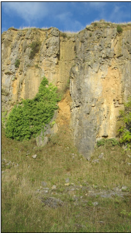
Pothole shaft in limestone.
