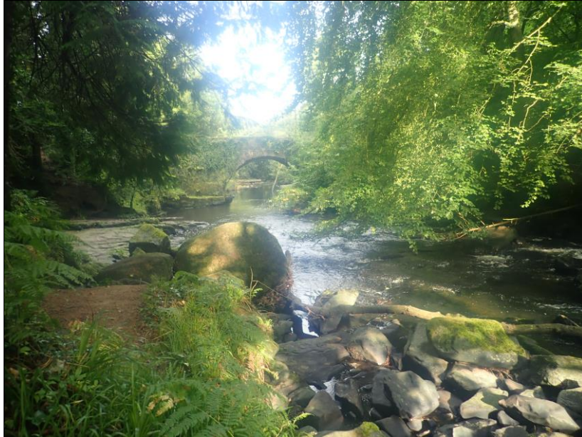
Clare Bridge, viewed from the southeast; see the huge sandstone boulders.
