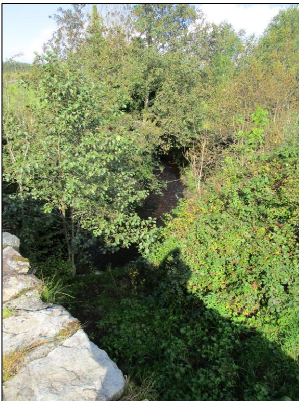
View upstream from Aghagrania Bridge.
