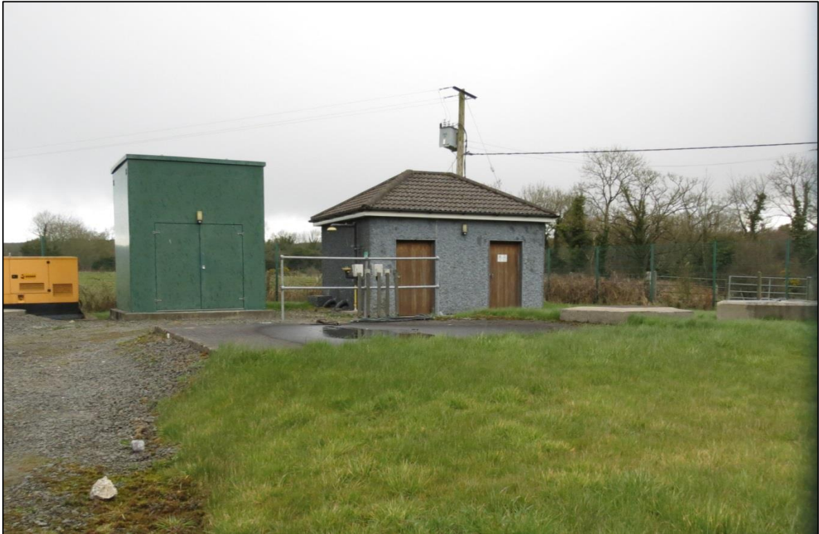
Pumphouse and works at Swan Public Water Supply Scheme. Clogh River to right near trees.
