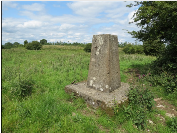
Trigonometrical (Trig) pillar sited on the rath enclosure just west of the “new” quarry.
