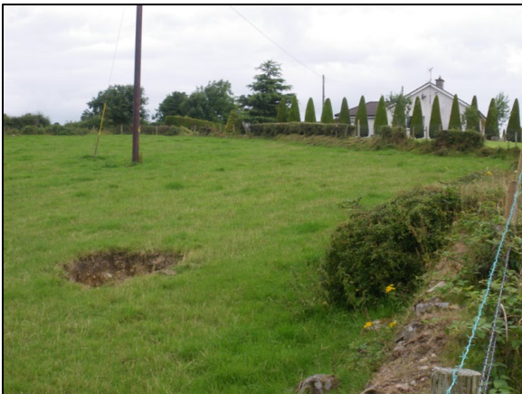
Collapse on site of historic shaft (see position on map).
