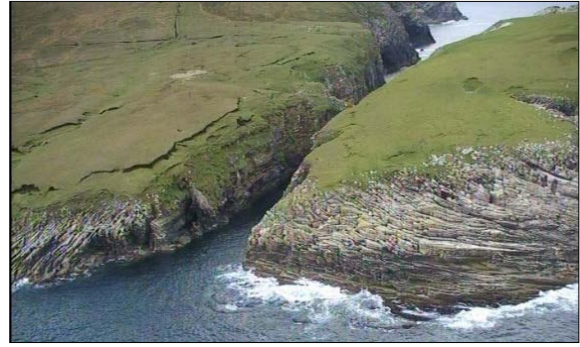
Location of Copper Mines at Geevraun. Horse Island (right) and the mainland (left). (Source: © Department of Communications, Marine and Natural Resources 2004)
