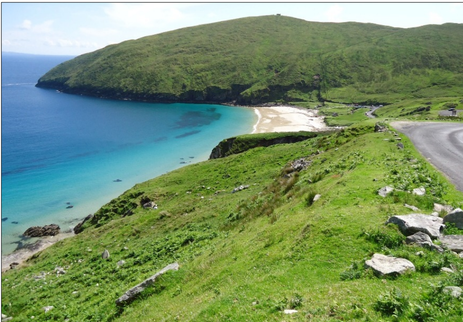
Vein extraction workings (from 1960s) below the road to Keem Beach. Vein quarry located to right of road.
