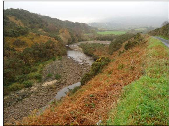
Looking upstream from road to Barnahowna (elevated road 300m north of bridge at Killateeaun).
