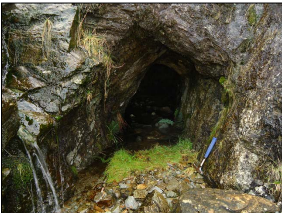
Entrance to mine. Adit turns c. 90° to left, 4m from mouth of adit.
