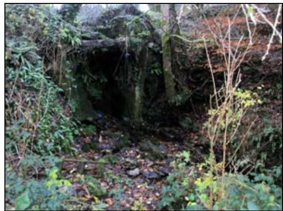
An unidentified structure with re-emerging stream from behind crude concrete wall.
