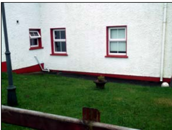
An air vent pipe in the front lawn of a cottage.
