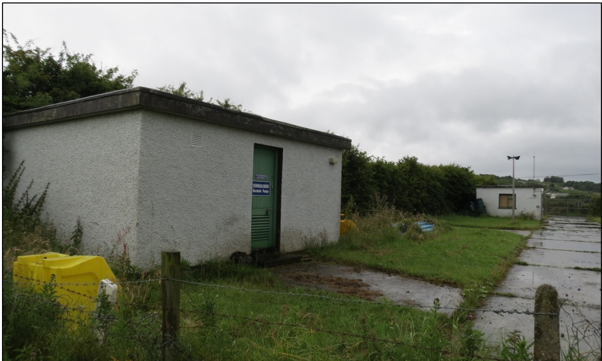
Pump house (housing sump for Gallery 1) at Carndonagh well field, looking west.
