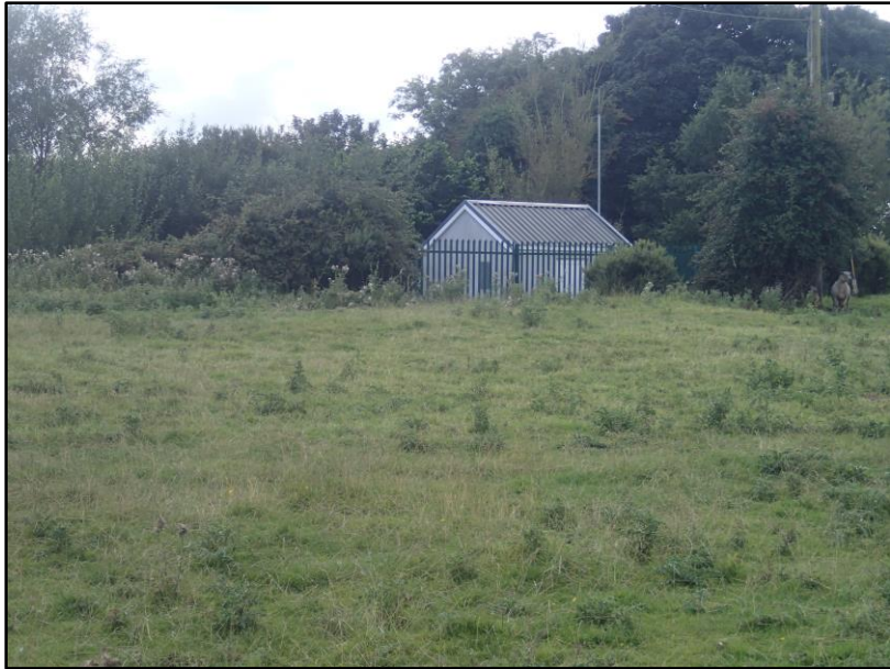
The compound housing the spring and adjacent pumphouse.
