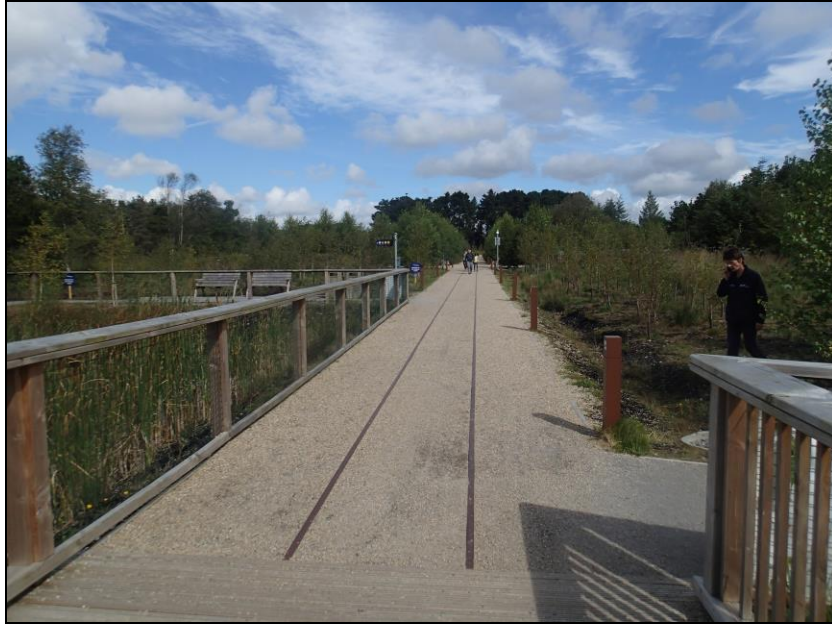
The entrance avenue to the Parklands, with the old railway preserved in the hardstand.
