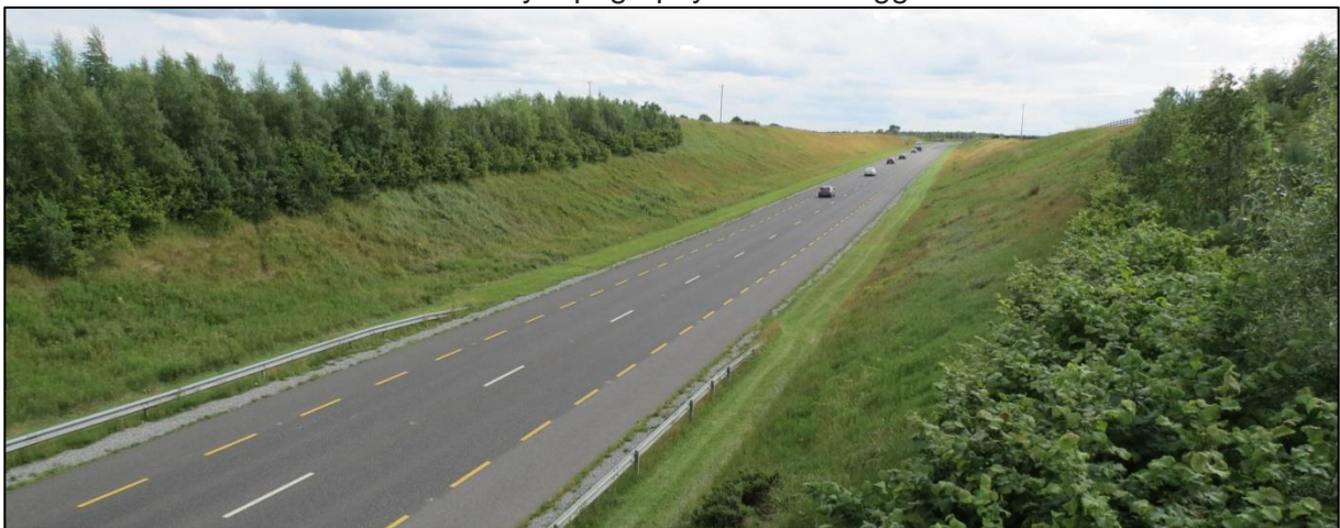
View SW from L2011 road bridge over N52 road (Mucklagh Bypass). Road excavations into Screggan Fan visible.
