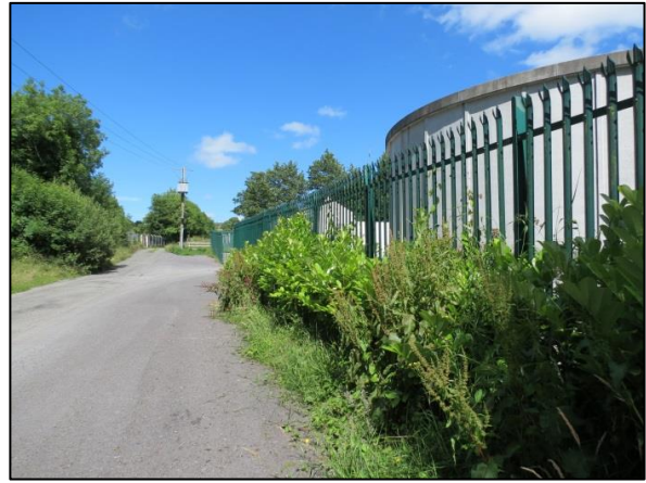
View NE along road. Heavey's Well far left side of road. Main works on right.
