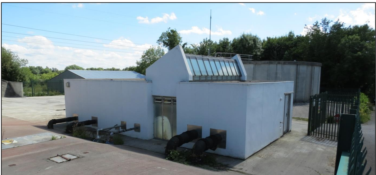
Main works site at Toberdaly. Pool Well in corrugated shed on rear-left.
