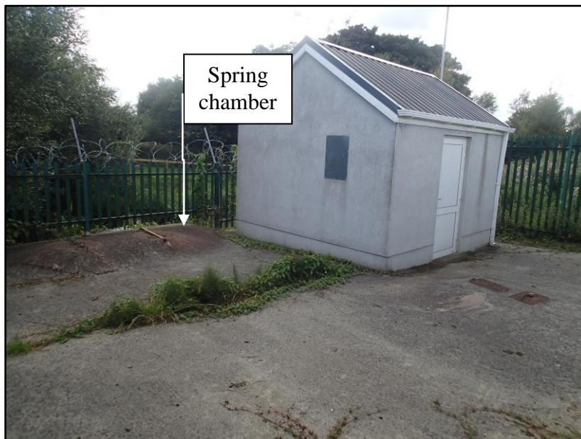
The pumphouse compound with the spring completely encased within the subsurface chamber.
