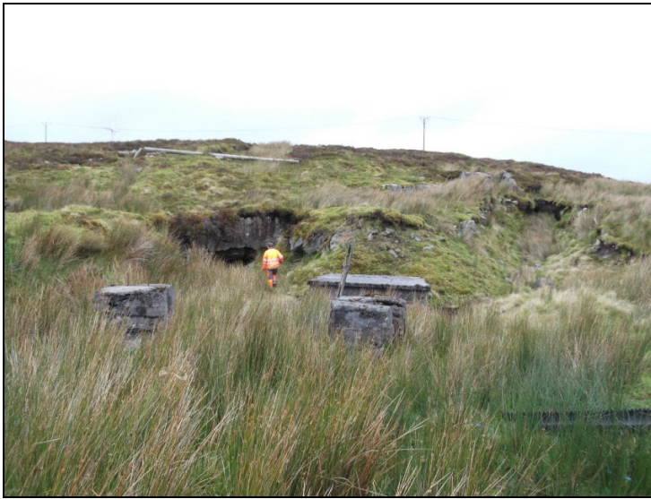
An adit, with adjacent concrete structures.
