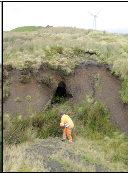
An adit visible in a surface cut.
