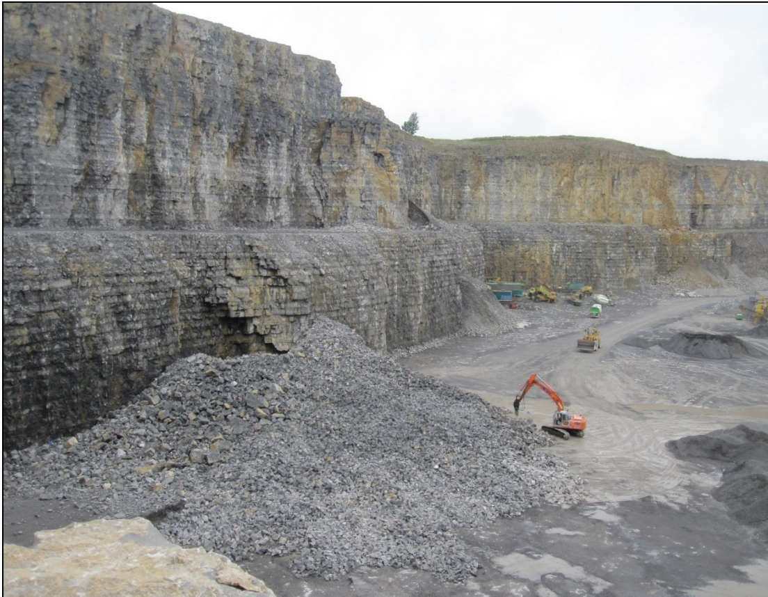
A view of Largin Quarry, looking southwest from the eastern side.
