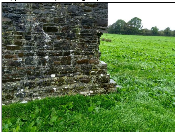
Copper chimney: missing stonework at base
