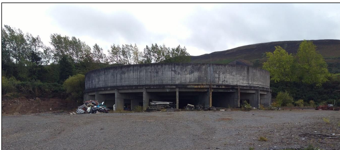
Large thickener, part of original processing plant.
