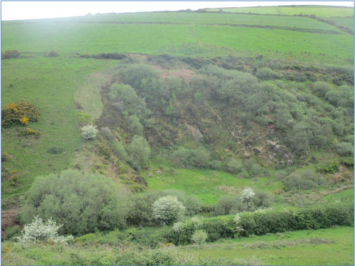
A view of the Reafadda Quarry from across the valley to the east.
