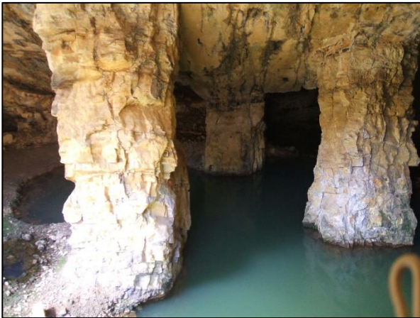
Cathedral Caverns - underground stopes exposed by opencast workings.
