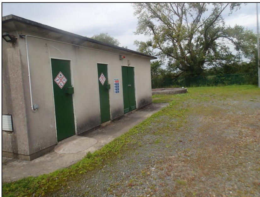
The pumphouse for the Tobernaloo Water Supply Scheme.
