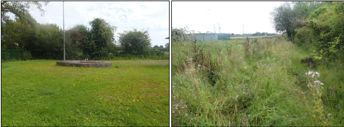
The chamber collecting water (left), and the overflow into the adjacent stream (right).
