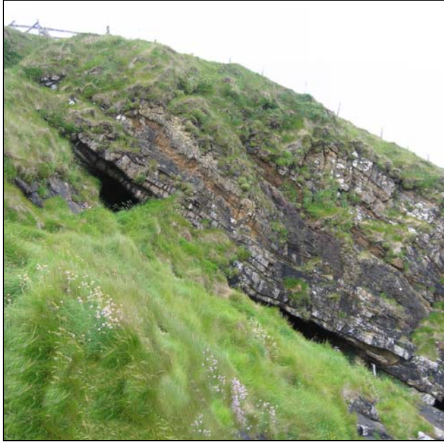
The mine adit entrances below the cliff path.
