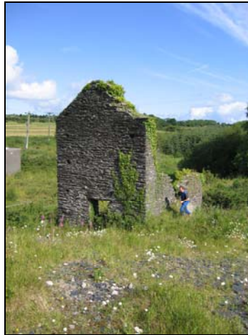
The water mill from the south.
