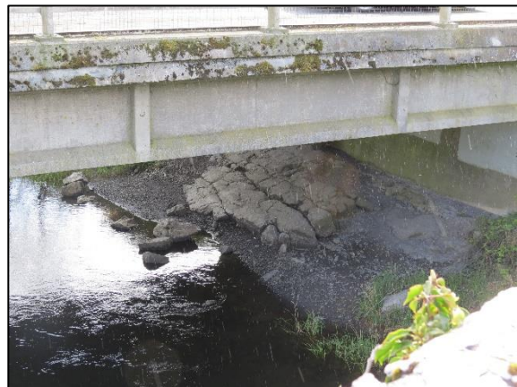
Limestone strata exposed on riverbank under new bridge.
