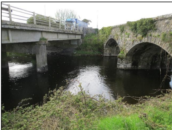
'New' and 'old' Ballinalack Bridge.
