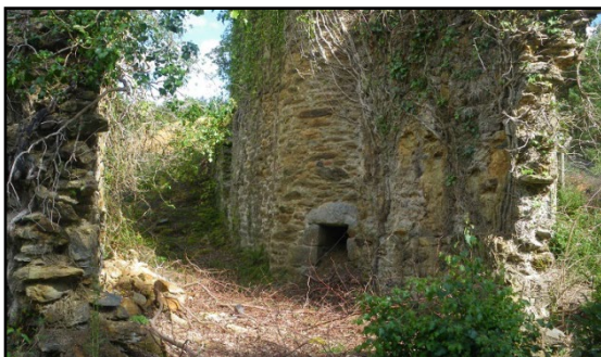
Left: Flue entrance at base of Baronet's Engine House chimney, revealed by recent site clearance
