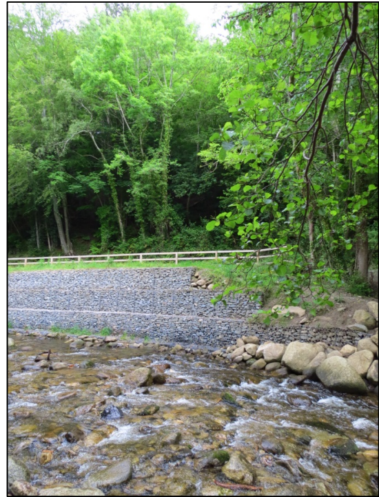
Stone reinforcements on NE riverbank river (between two wooden bridges in Knocksink Wood).
