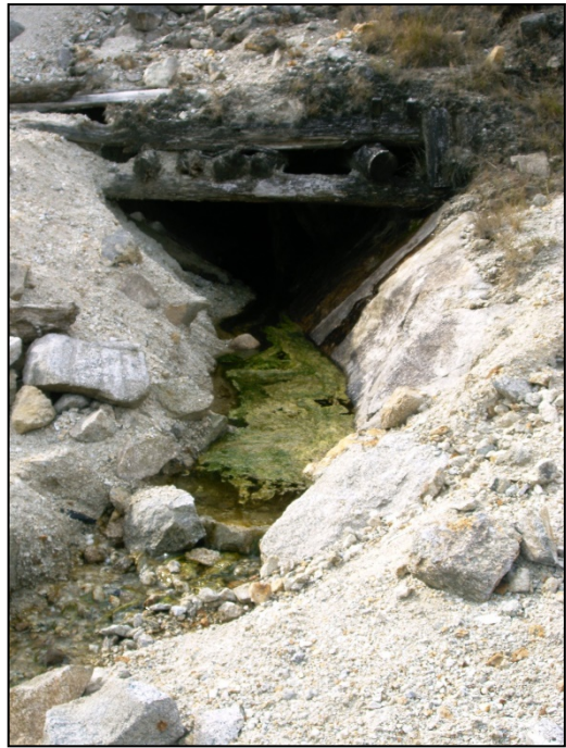
3 rd Adit on Foxrock lode, July 2014, showing almost complete closure of entrance by siltation. Photo on right is from 2007.
