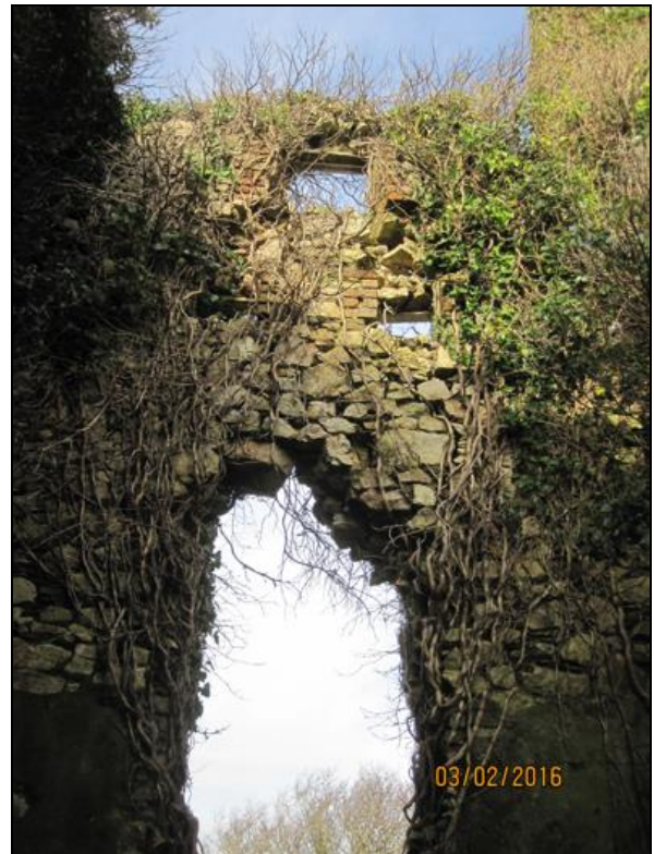
Precarious masonry in need of consolidation and conservation work.
