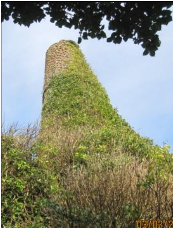
The brick top of the chimney survives better than many such structures.
