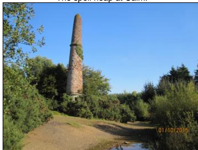
One chimney with brick top.
