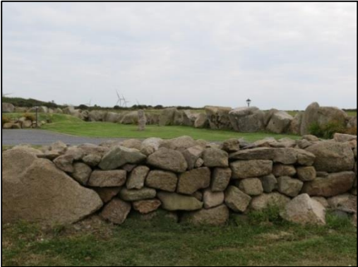
Granite walls at Carnsore. Wind turbine in background.
