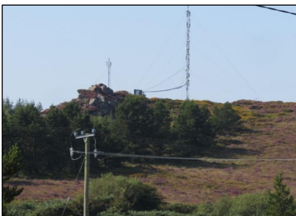
Carrickadee Rock tor with telecoms mast.
