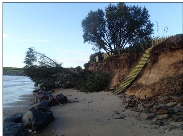
Erosion at the southern end of the site.
