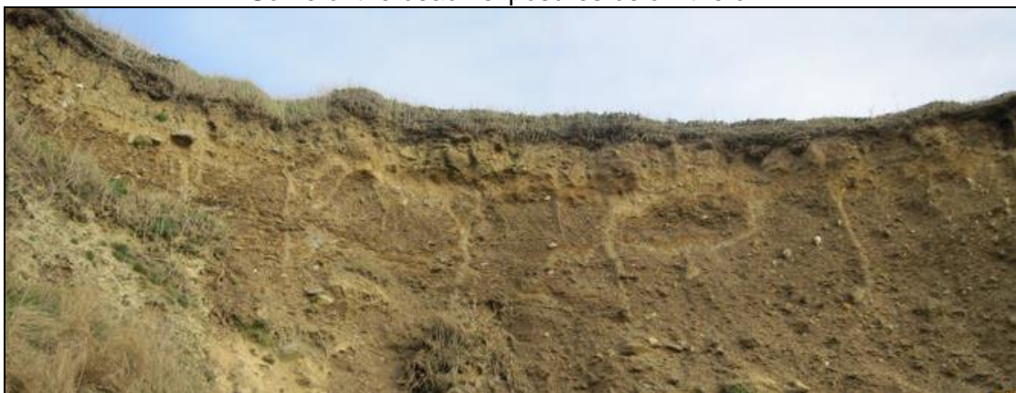
Infilled till cracks in the cliff top at Loftusacre.
