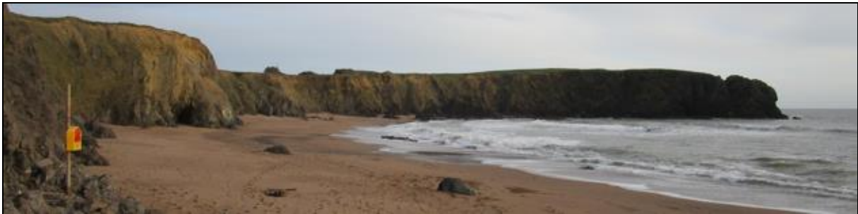
The section on Petit's Bay from the western beach access track. Note the warning sign.
