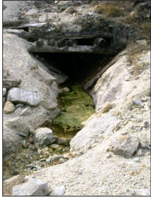
3<sup>rd</sup> Adit on Foxrock lode, July 2014, showing almost complete closure of entrance by siltation. Photo on right is from 2007.
