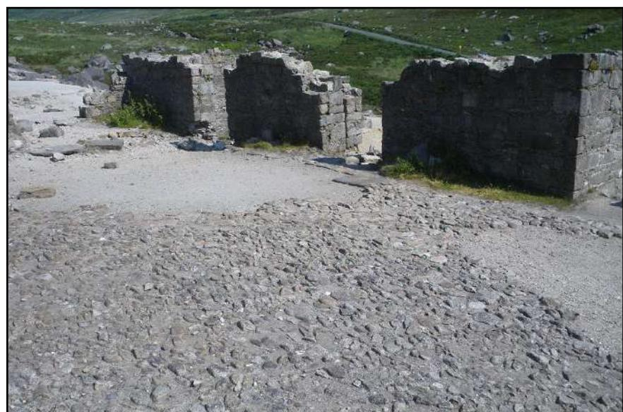
Dressing floor where ore was 'cobbed' prior to crushing by stamps.
