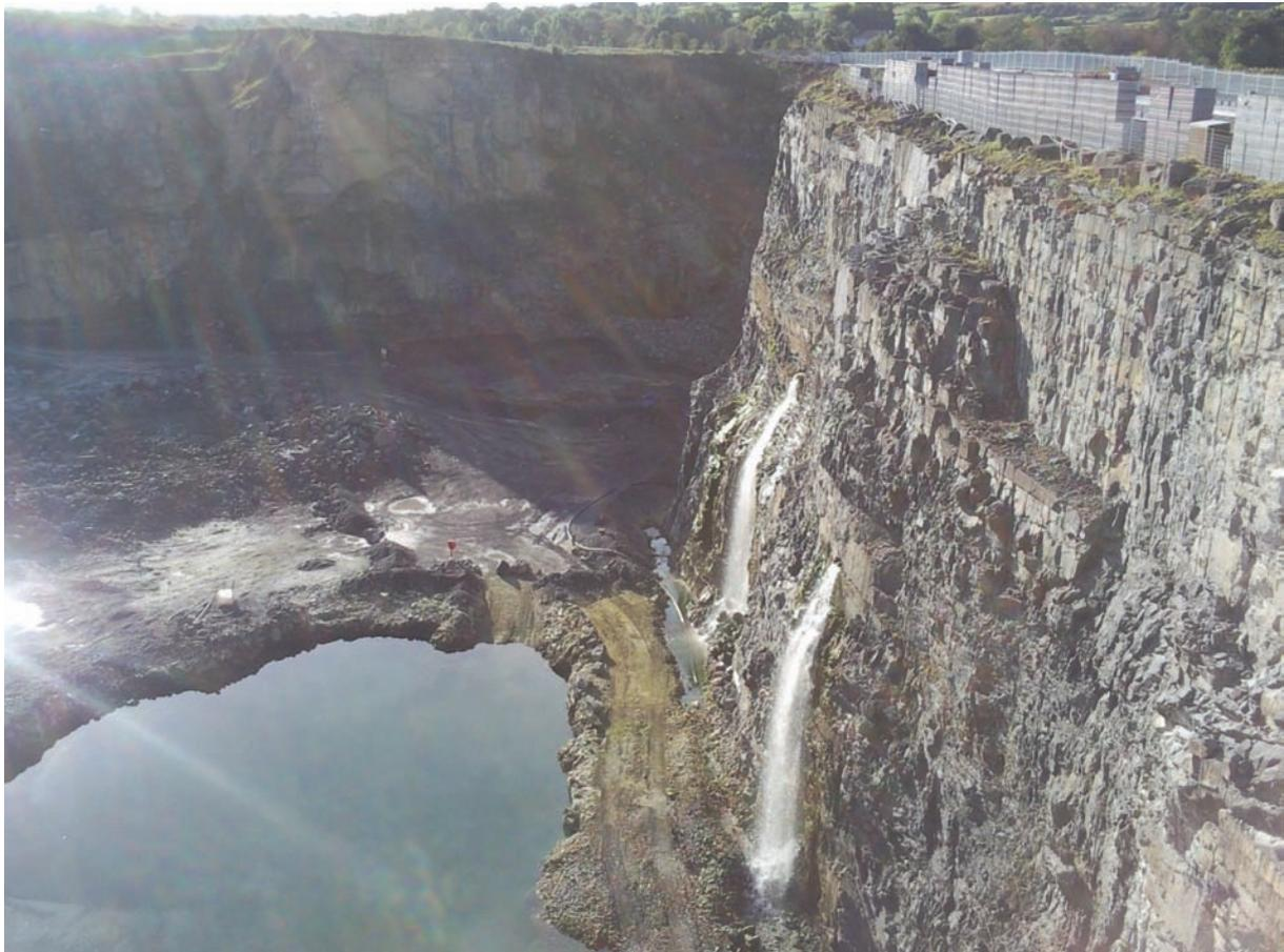
Figure 8.15 Pure bedded limestones with large water bearing conduits at two different depths (LeCarrow, County Roscommon). (*Photograph by Caoimhe Hickey.*)
