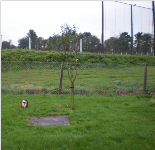
Photo 4: BH2 Steel Manhole Cover
