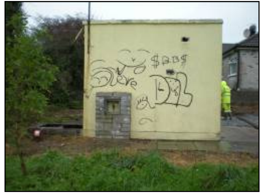
Photo 3: Pump House and the BH1 Concrete Manhole at the rear
