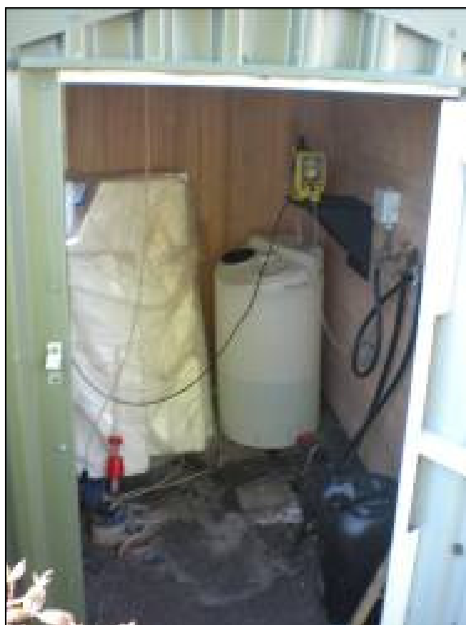
Photo 4: Chlorine system in the pump house
