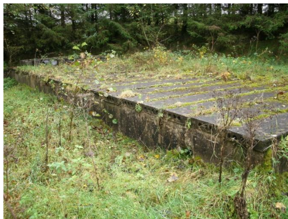
Figure 3 Main Chamber at Mountnorth Spring, concreted over (Donal Crean (OCM))
