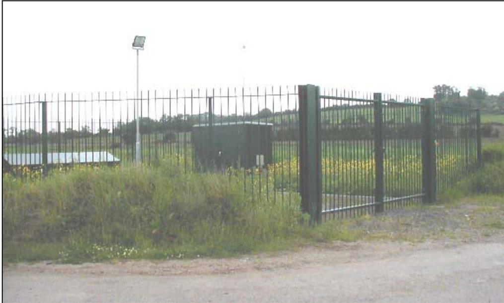
**Figure 1: Production well 2 (PW2), showing the concrete platform, railings, well-head protection cabin and pump-control housing.**
