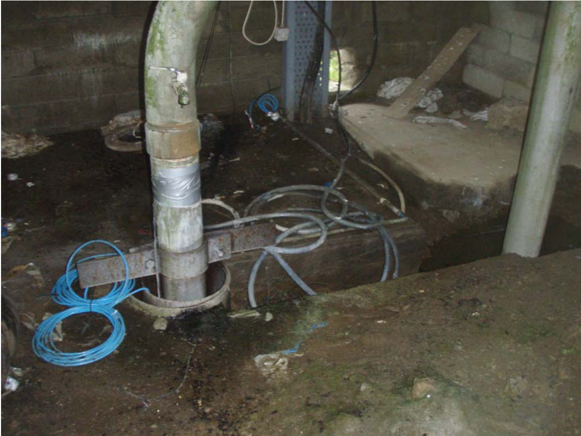
Plate 2 Detail of borehole PW2.
