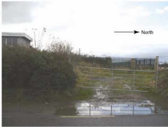
Photo 1: Entrance to Ballymakenny GWS
