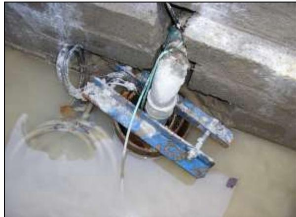
**Figure 3** Mouth of borehole PWSBH01 inside borehole chamber.
