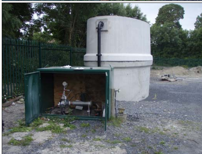
Photographs of Meelick Borehole showing the well head and the large storage chamber used for augmentation to Ballyroan WS.
