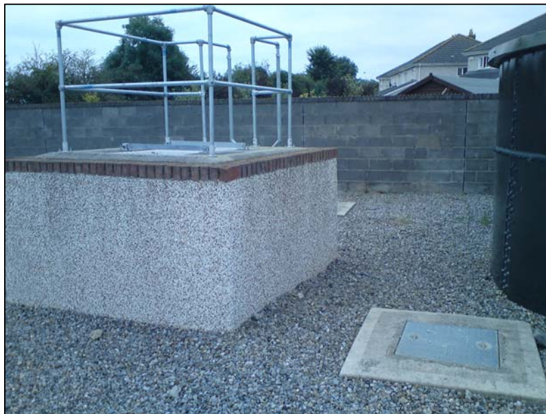
Photograph 1 Borehole cover and adjacent treatment works
