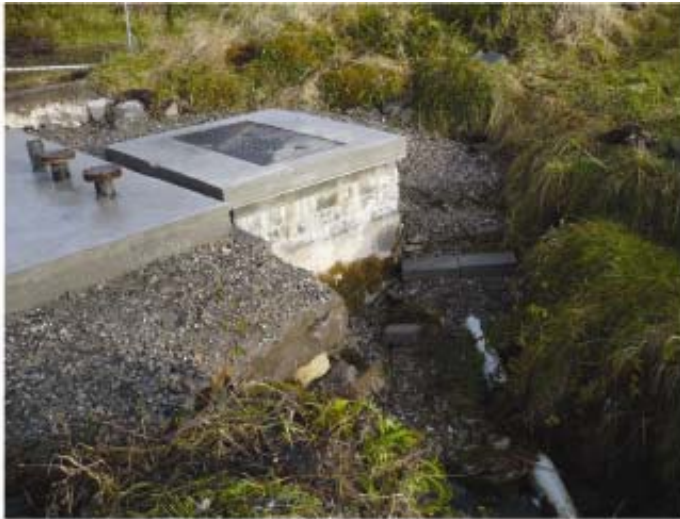
Photo 1: Spring 1 with overflow pipe
