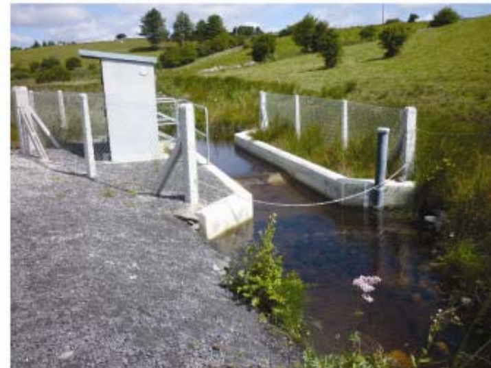
Photo 4: EPA weir and gauging station
