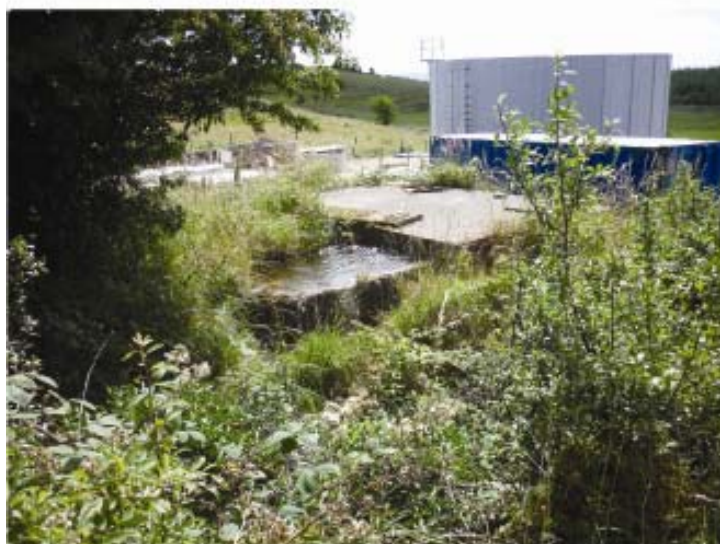
Photo 6: "Stream box" damming up stream (new reservoir in background)
