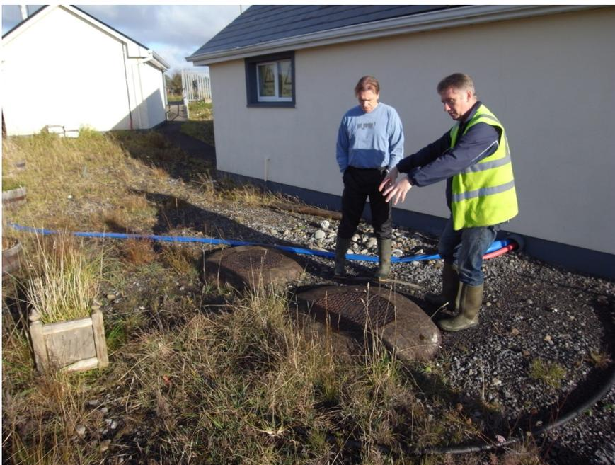
Caisson wells collecting 'deep' water from apparent upwellings of groundwater from the limestone bedrock beneath
