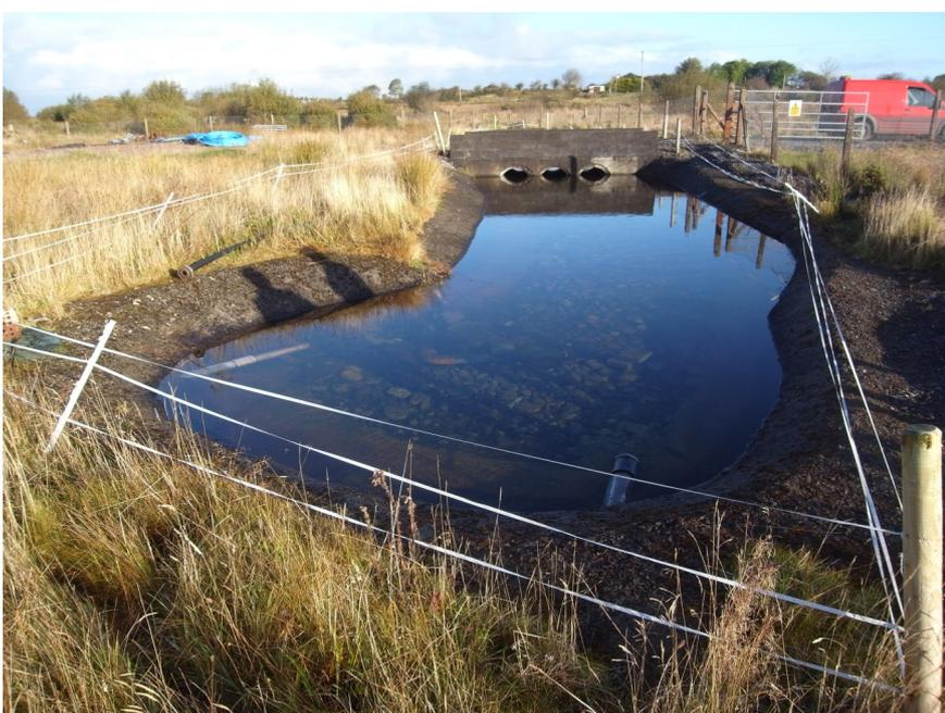
Killaturly GWS pond which collects groundwater from two gravel springs (inflow pipes visible below water level)
